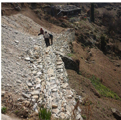
Stones support the mountain slope where the new classrooms will be.
