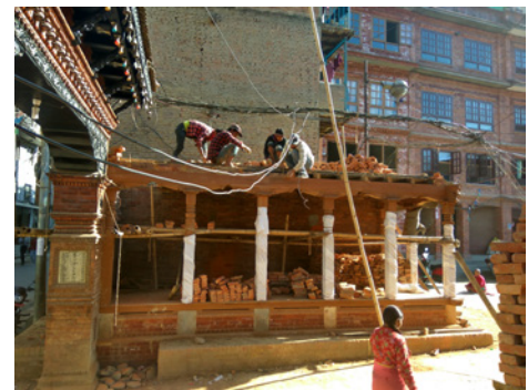
Construction on the pati in Old Patan continues.
