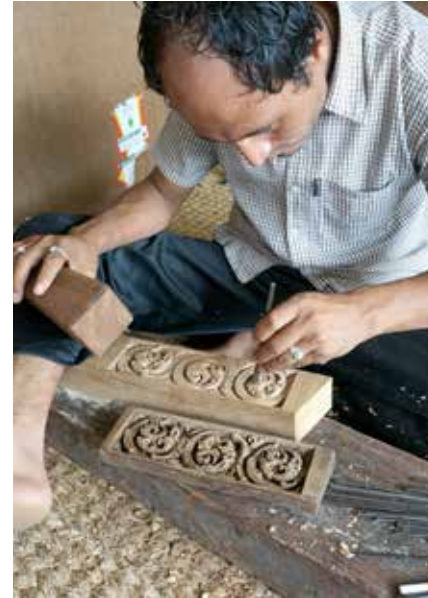
Manimandapa Pati South | May 29 & June 01, 2016 A window bracket of the south pati is being replicated including cornice ( kulah ) and window assembling.
