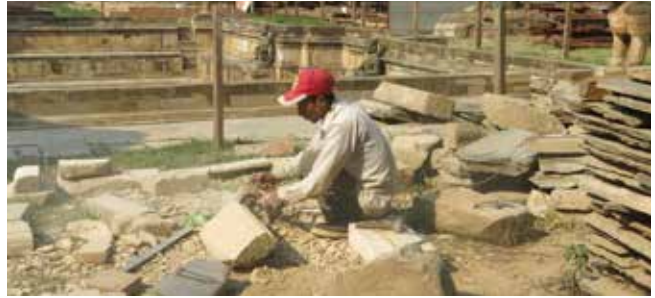
Manimandapa Pati South | Carpenter adding tenon to the repaired pillar. Stone mason chiseling and sizing the stone for making quarter round ( nagol ) on the top edge.
