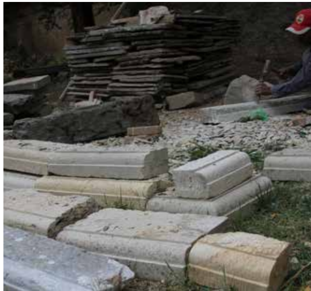
Manimandapa Pati South | May 05, 2016 Stone mason making quarter round ( nagol ) by chiseling the stone on top edge.
