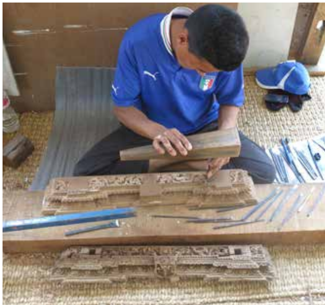
Manimandapa Pati South | April 25 & 29, 2016 Woodcarvers replicating the missing parts of the windows of the Pati such as pillar and kulah .
