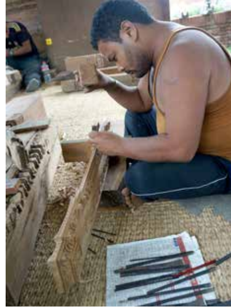
Manimandapa Pati South | May 24, 2016 Carpenter repairing and retrofitting the capital ( meth ) of the column using the traditional material wood including bamboo pegs. Woodcarver replicating the window cornice kulah .
