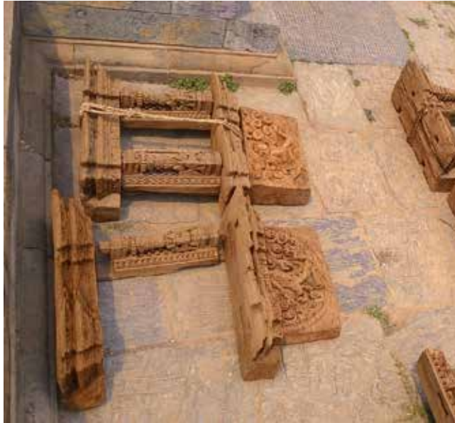
Manimandapa Pati South | April 06 2016 The windows that were cleaned and stored were assembled to identify the missing parts for replication and repair work.
